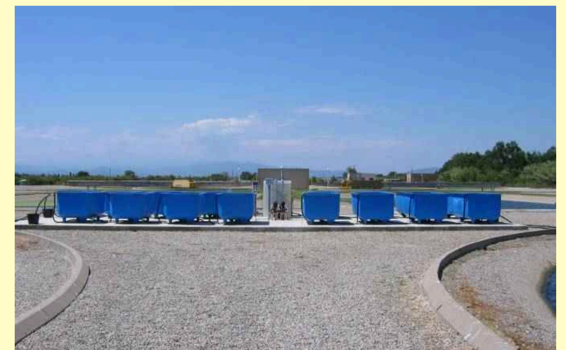
STP Empuriabrava, Costa Brava, Spain Very low loaded activated sludge (oxidation ditch) Full-scale Daphnia ponds "Understanding the full scale process" Food web studies, harvesting of Daphnia
